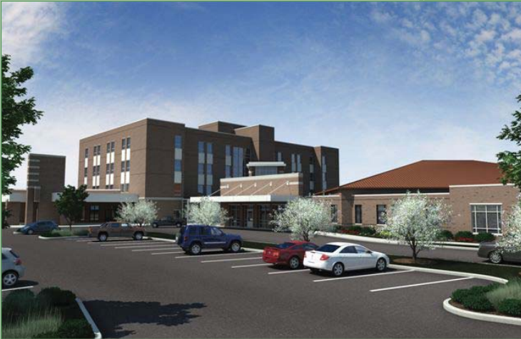
The Exterior of the Building at completion
