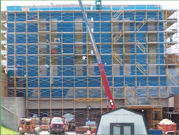
Phase 3: Waterproofing North elevation prior to the laying of new brick
