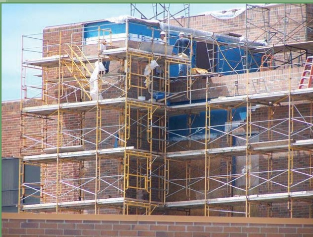
Phase 4: New Brick Northeast corner with new brick nearly complete
