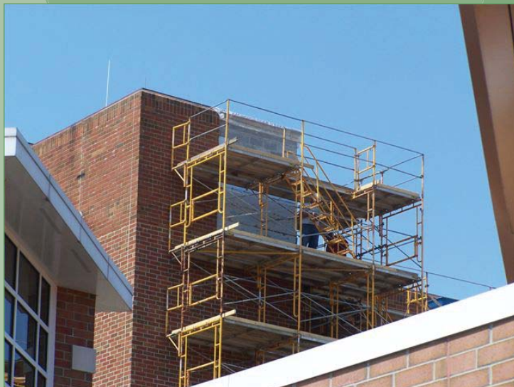
Phase 2: Demolition Begins Center East Tower, April 15
