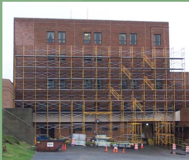
Phase 1: Scaffolding Began the week of March 15
