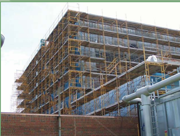
Demolition beginning on the west elevation in early June
